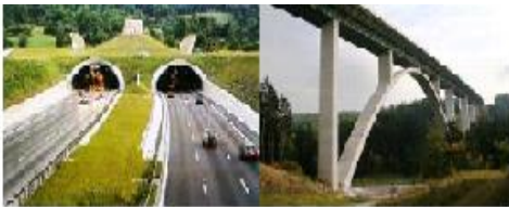
Autobahn tunnel (left) and valley bridge (right)
